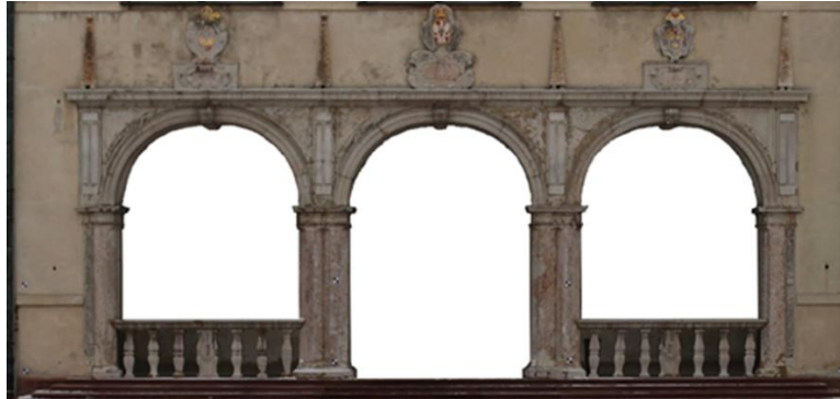
Fig. 6. Fragment of the orthophotomap of the Bishops' Palace wall, with GSD 3mm ( Brożyna & Kabata, 2016 )
