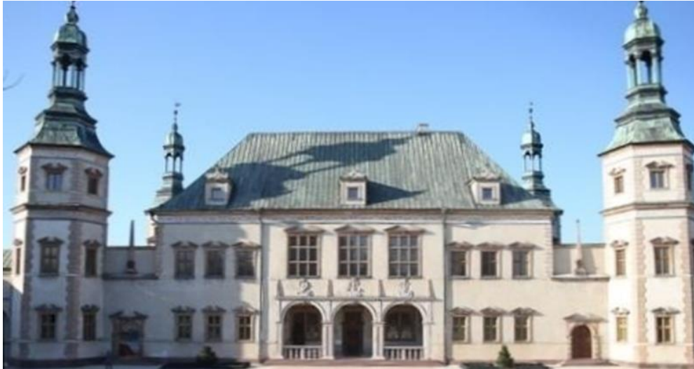
Fig. 1. Photo of the Palace of Kraków Bishops in Kielce
